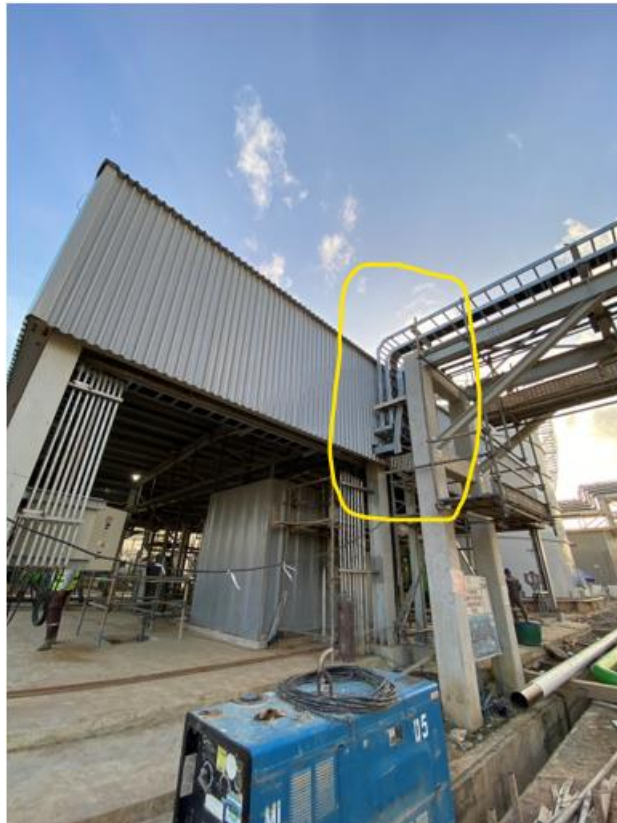
Gambar 4. 12 Keadaan Aktual di Drainage Pump Station
