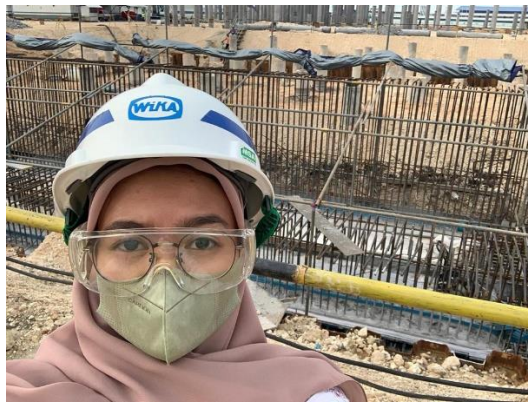
Gambar 5. 24 Pengamatan Progress RO Building
