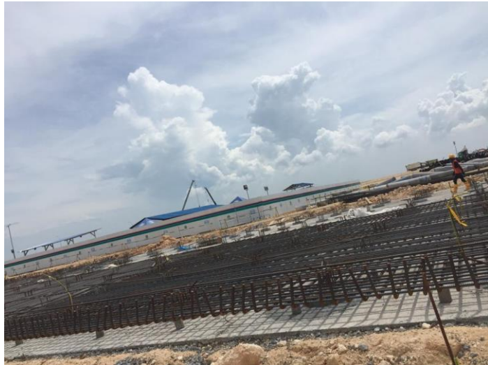
Gambar 5. 25 Progress Pekerjaan Area GDMF Tank
