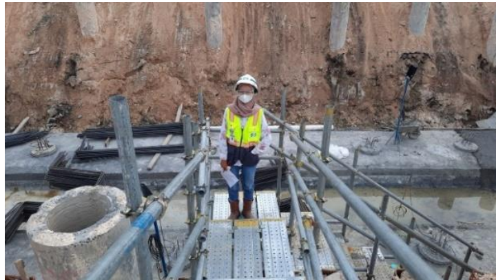
Gambar 5. 21 Pengamatan Progress RO Building
