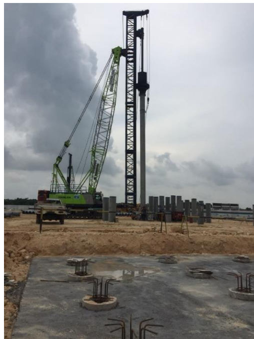
Gambar 5. 22 Progress Pemasangan Pre-Sedimentation
