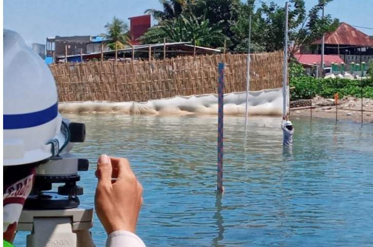
Gambar 3.6 Monitoring Sattlement Plate (Sumber: PT. Wijaya Karya, 2022)
