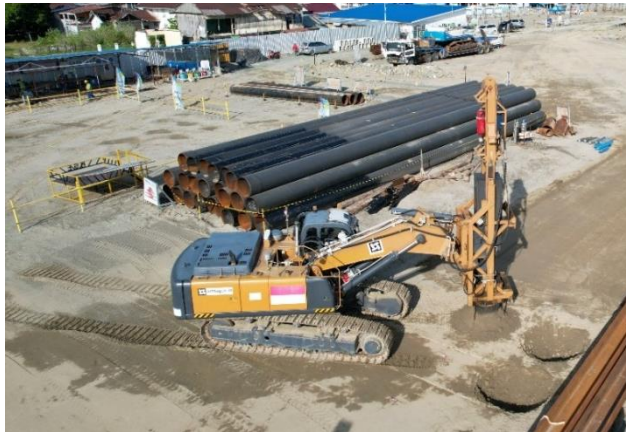
Gambar 3.5 Dynamic Compaction (Sumber: PT. Wijaya Karya, 2022)
