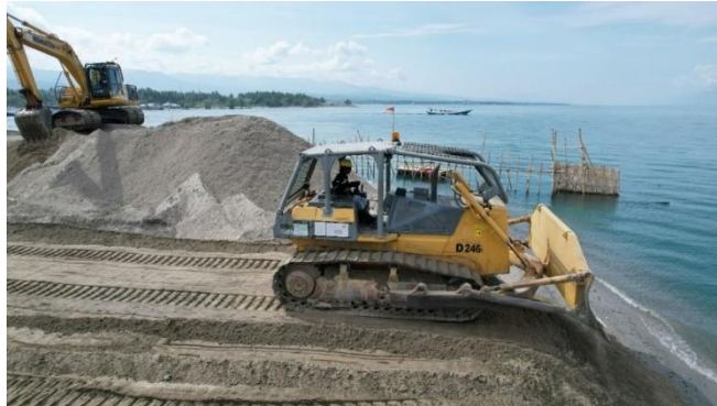
Gambar 3.1 Bulldozer Komatsu-D85E-S5 (Sumber: PT. Wijaya Karya, 2022)
