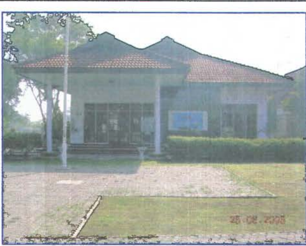
Gambar 4.1 Tampak depan kantor Plant Watudakon
