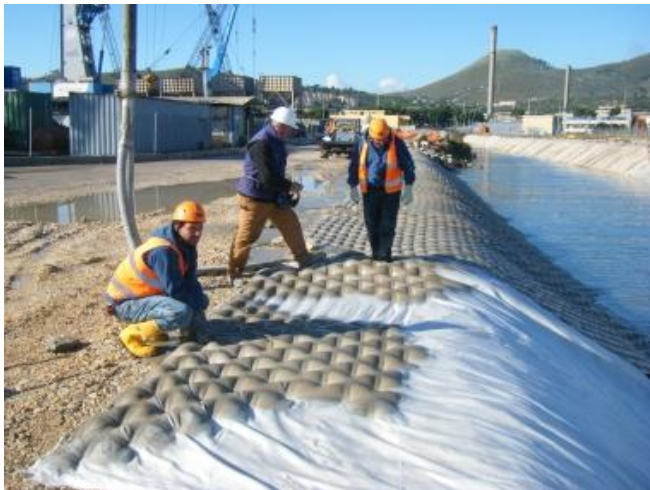
Gambar 1.5 Concrete Mattress (Sumber: www.geosintex.com )
