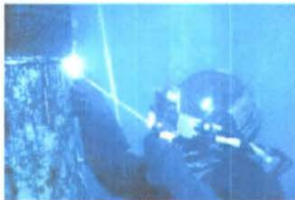
Gambar 2.1. Manual SMAW Wet Welding (Joshi, 2000)
