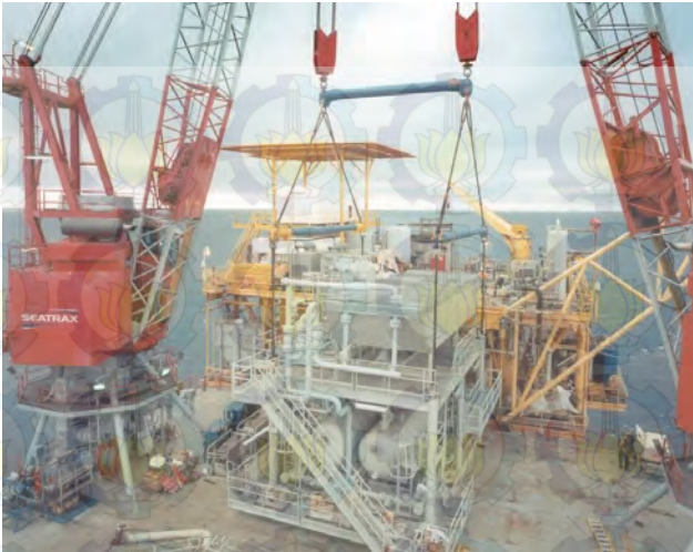
Figure 2.4 Liftboat Perform Crane Operation ( http://www.semcollc.com/200_ton_tandem_lift.jpg )
