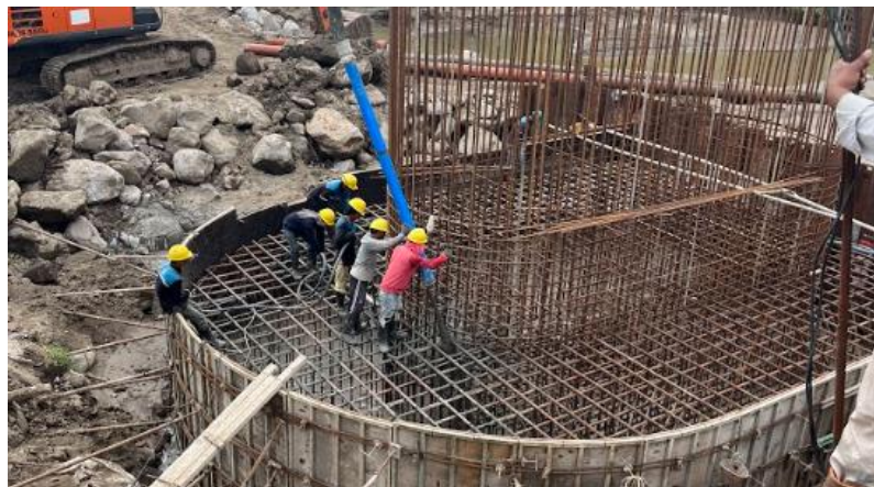
Gambar 2. 24 Proses Pengecoran Footing Pilar 3
