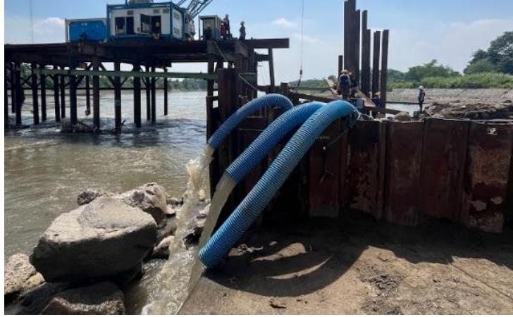
Gambar 5. 26 Dewatering Area P-3
