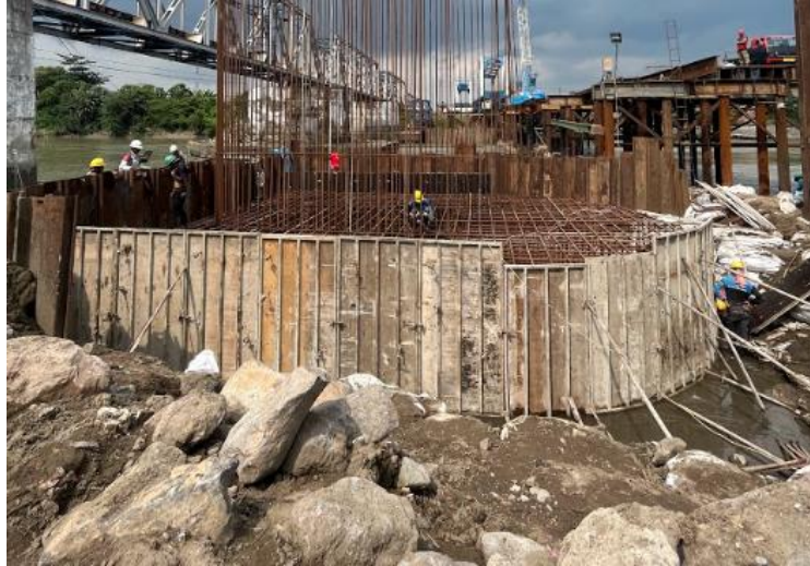
Gambar 5. 29 Pemasangan Bekisting Footing Pier P-3
