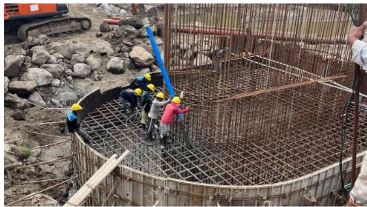
Gambar 5. 30 Pengecoran Footing Pier P-3
