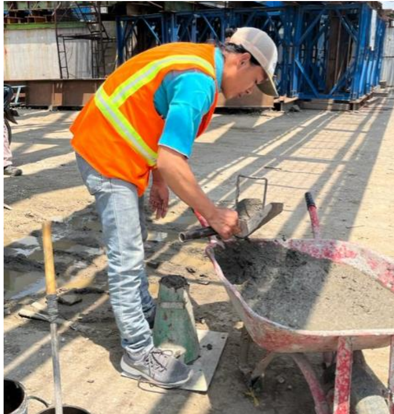
Gambar 5. 40 Proses Uji Slump Beton Pier
