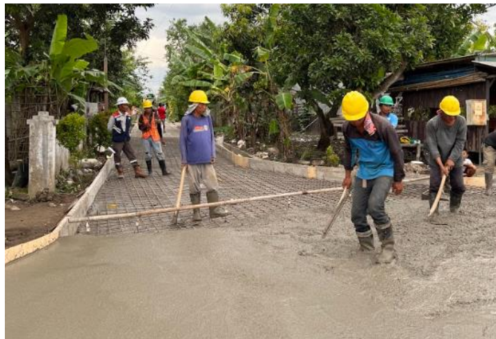
Gambar 5. 49 Pengecoran Rigid Pavement
