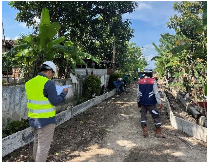
Gambar 2. 40 Bekisting Rigid Pavement
