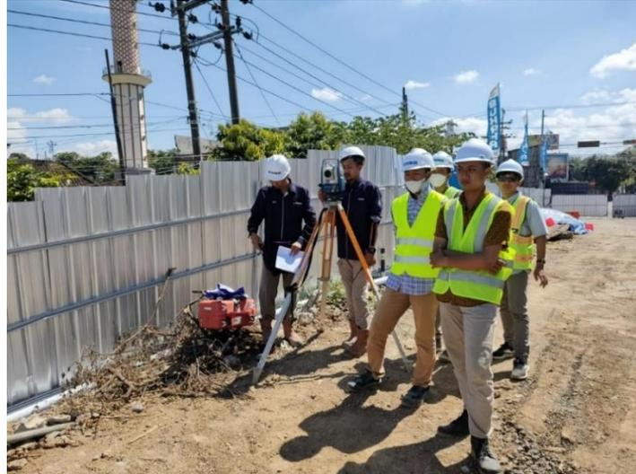
Gambar 3.5 *Setting Out Posisi Pile*
