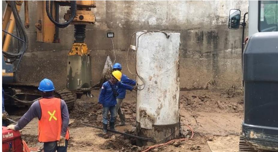
Gambar 3.9 Pemasangan *Casing Temporary*
