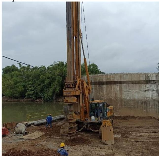
Gambar 3.6 *Boring Bore pile*
