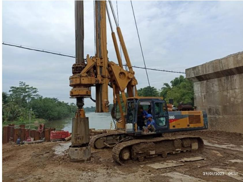
Gambar 3.7 *Drilling Bore pile*
