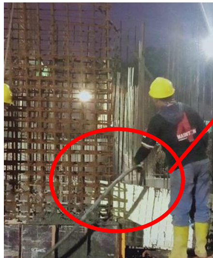
Gambar 4.44 Pengecoran Shearwall
