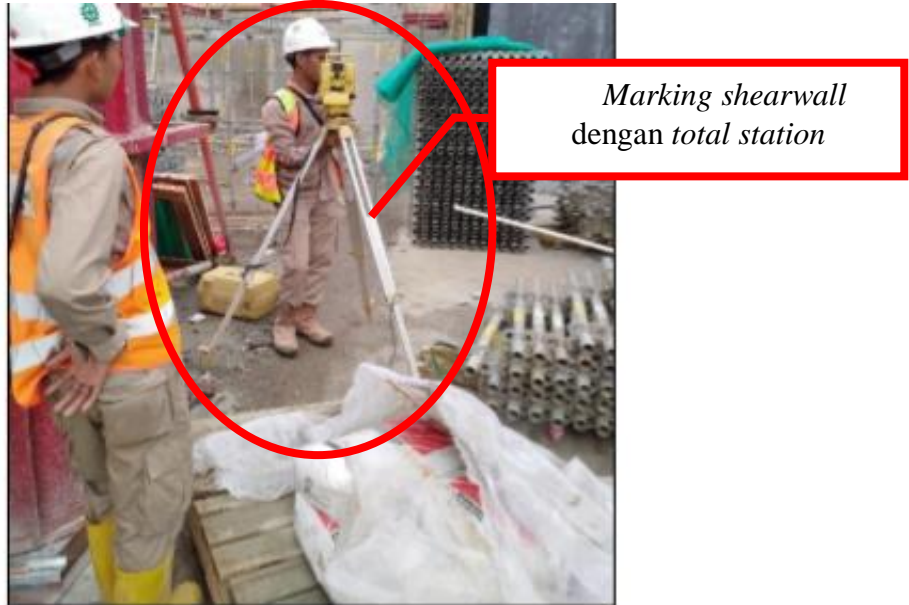
Gambar 4.35 Marking As Shearwall
