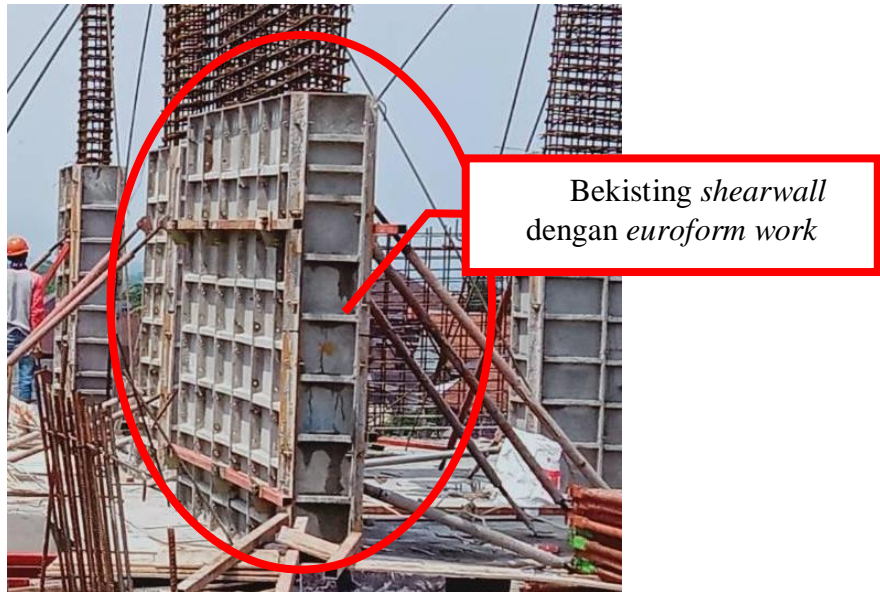
Gambar 4.40 Bekisting Shearwall
