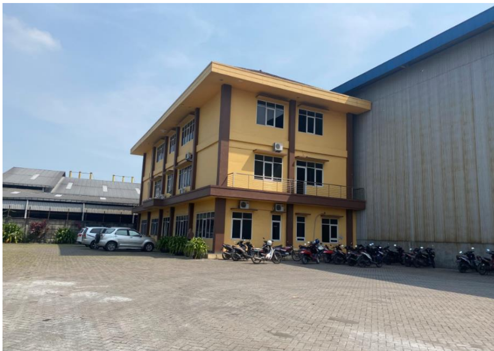
Gambar 2.3 Kantor PT. Perwira Indo Wire
