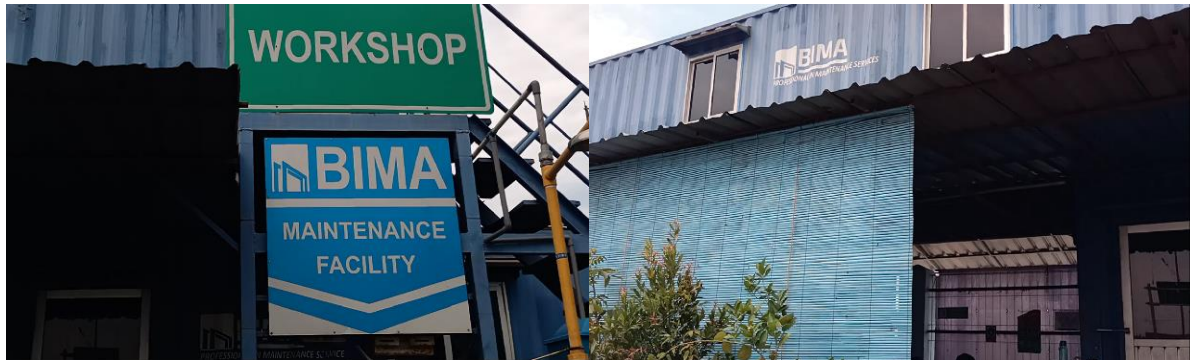
Gambar 2. 6 Site maintenance facility PT BIMA di Pelabuhan Nilam
