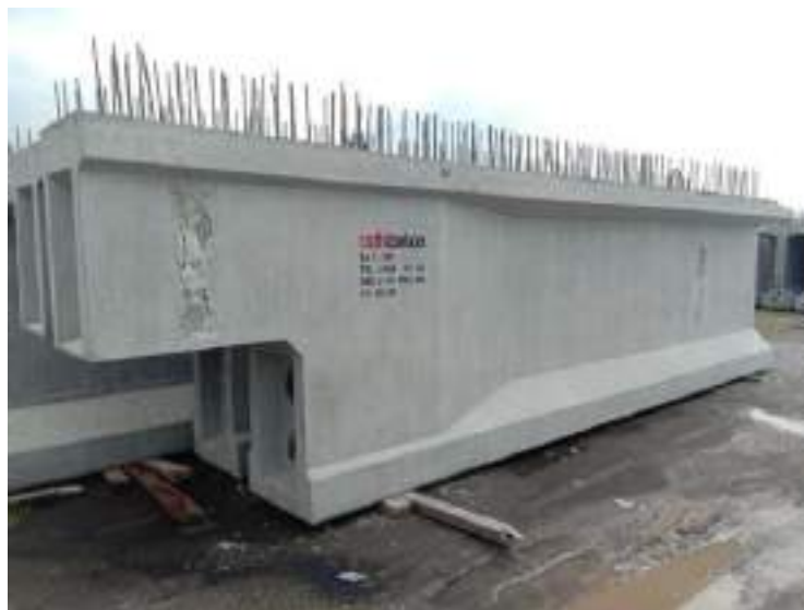
Gambar 2.4 PCI Girder
