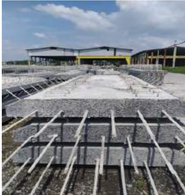
Gambar 2.5 Half Slab
