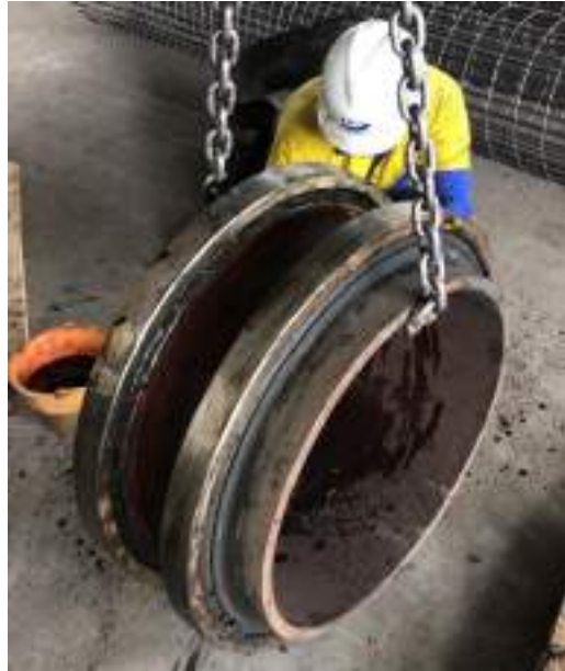
Gambar 4.37 Bearing Mesin Cage Forming Macet
