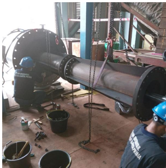
Gambar 4.13 Condensate Extraction Pump
