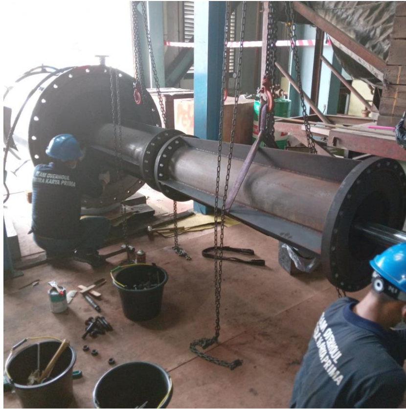
Gambar 4.27 Condensate Extraction Pump
