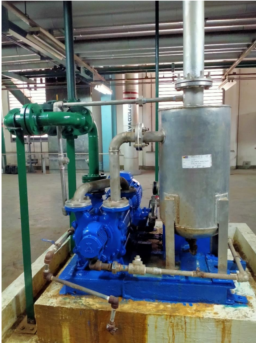
Gambar 4.33 Priming Vacuum Pump
