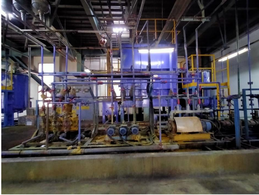
Gambar 4.29 Ferrous Pump
