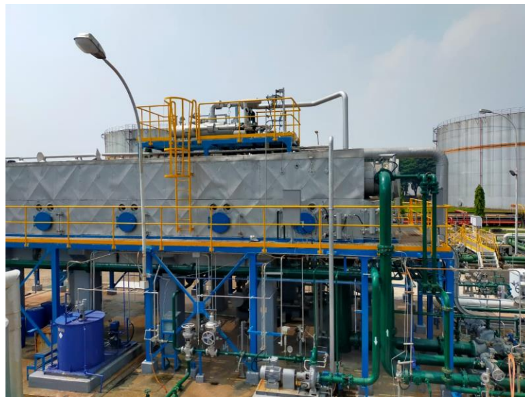
Gambar 4.15 Flash Evaporator
