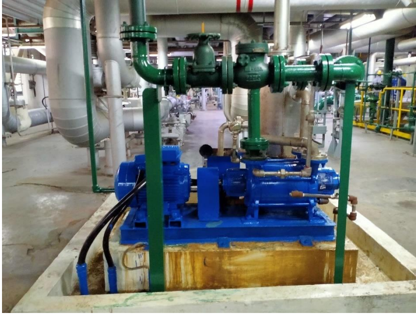
Gambar 4.32 Priming Vacuum Pump
