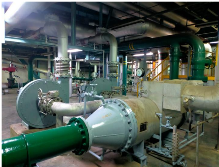
Gambar 4. 28 Gland Steam Condenser
